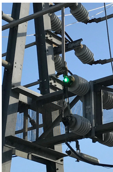
Figure 3: Substation switch identified by DFA
